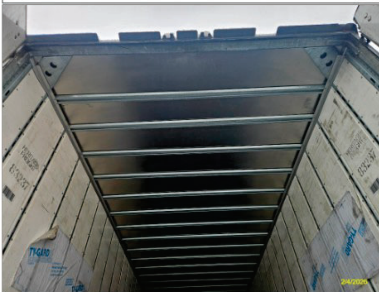
Trailer inner ceiling
