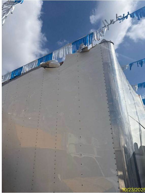
Description: Damage Area - From Right Angle
