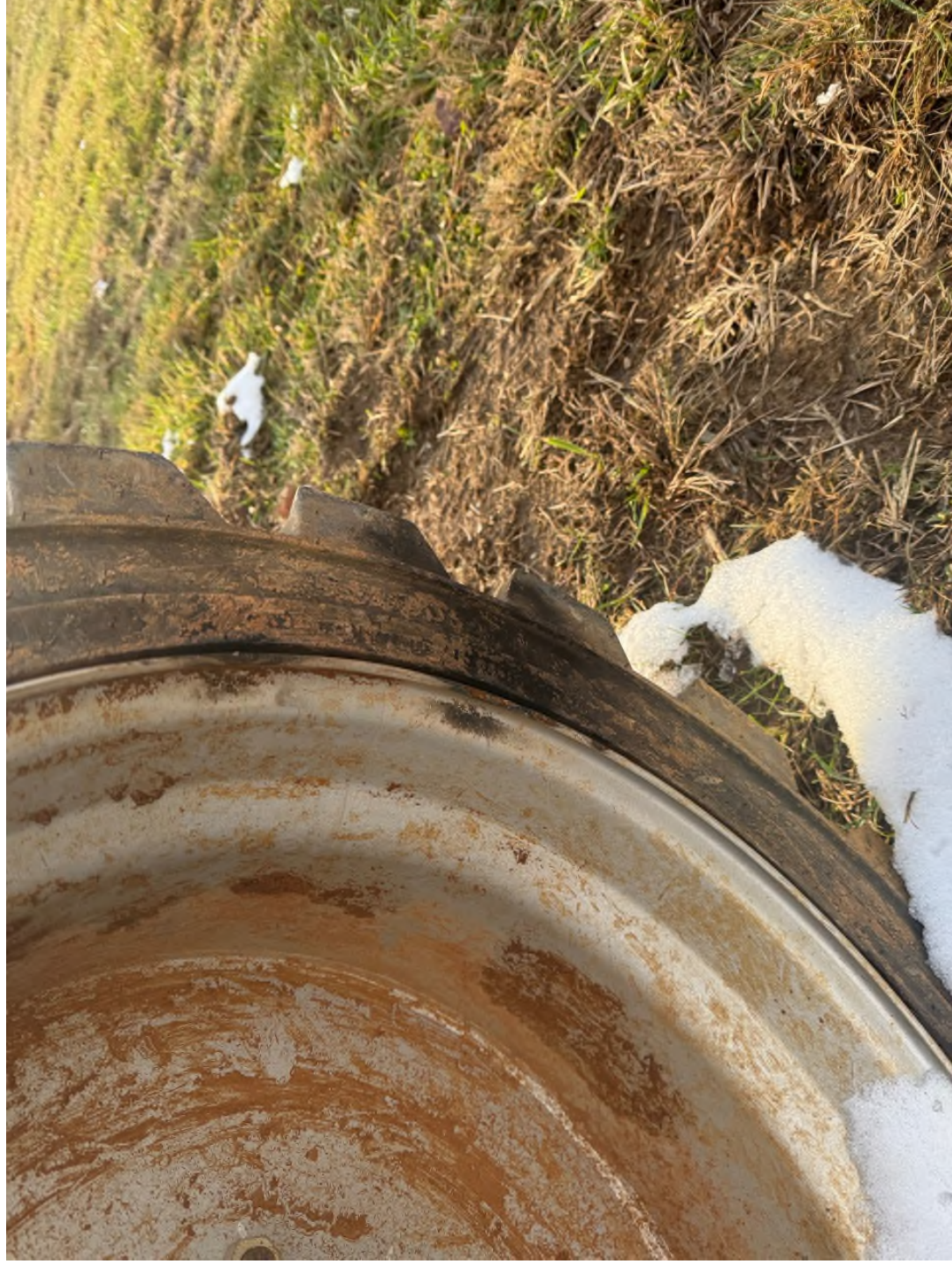
Damage overview photos.
