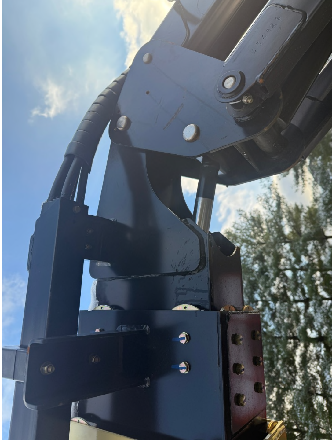
Damage overview photos.
